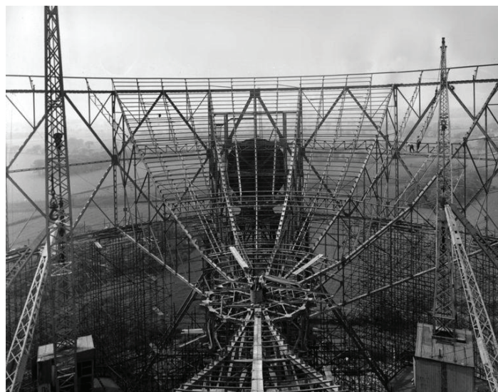
The Jodrell Bank’s Mark I radio telescope being built.
