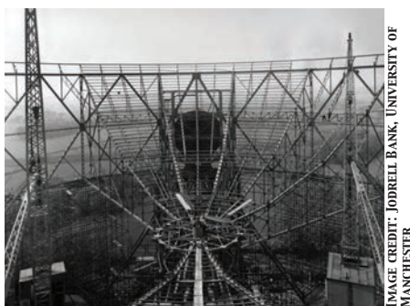
The Jodrell Bank's Mark I radio telescope being built.
